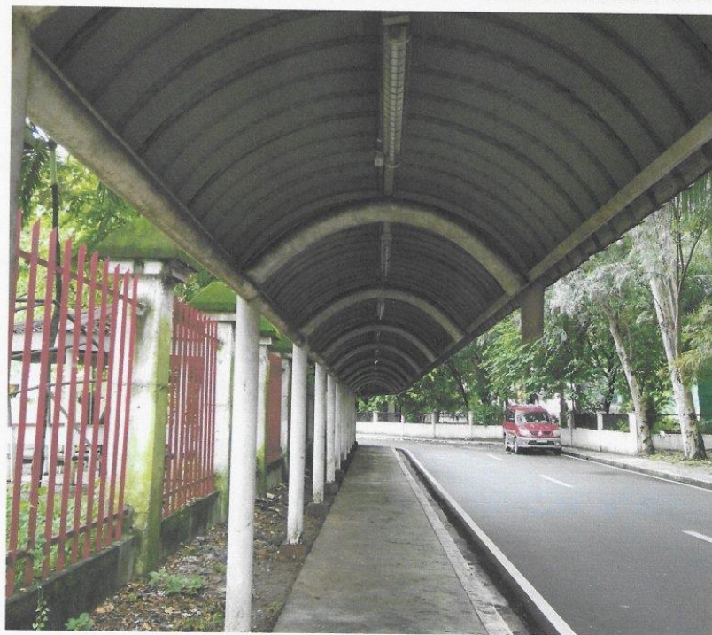
COVERED PATHWAYS AT MAIN CAMPUS
