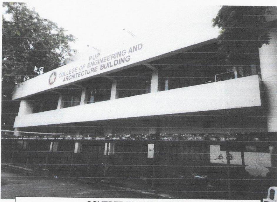
COVERED WALKS AROUND COLLEGE OF ENGINEERING AND ARCHITECTURE BUILDING
